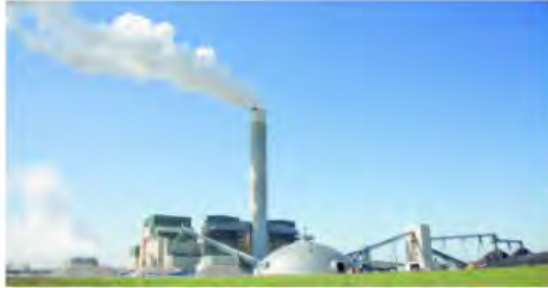
Decarbonize Energy Sources Prairie State, Peaking Power
